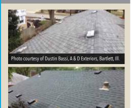
THE FIX: Keep exhaust vents high on the roof where they were designed to be; install soffit, undereave or edge-of-roof style intake vents. Using exhaust vents as intake vents increases the chance of a roof leak and weather infiltration because they are designed to be 2-3 feet from the peak of the roof.
