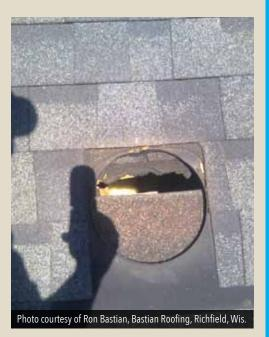
THE FIX: Cut the vent hole according to the manufacturer's installation requirements to maximize the vent's Net Free Area and to provide the attic with necessary airflow. RC
