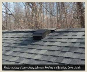
THE FIX: Don't mix any two different types of exhaust vents (ridge vents, power fans, wind turbines, roof louvers or gable louvers) so as to avoid short-circuiting the attic ventilation system. Short-circuiting reduces the efficiency of the system and could result in weather infiltration.
