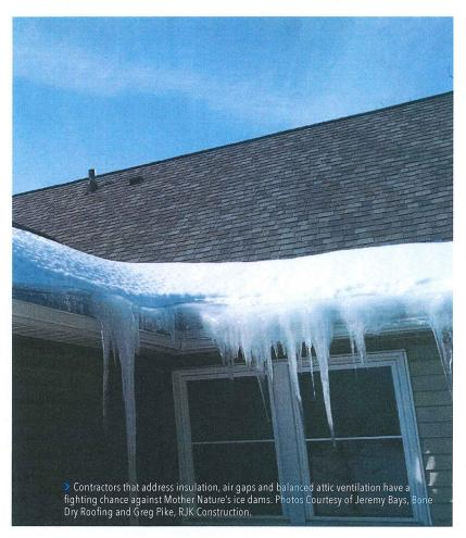
primarily due to uneven roof deck temperatures. It usually starts near the peak where it's warmest and refreezes when it reaches the lowest, coldest section of the roof. Any additional snow melt in the next hours or days runs into the ice dam – and the real trouble begins.
