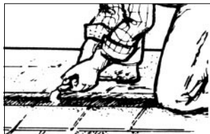
5. Cut through shingles to roof sheathing with utility knife.
