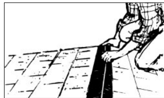
2. Snap chalk line along centerline of peak.
