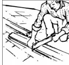
7. Extend FilterVent past ends of slot to full length of ridge. Cut final section.
