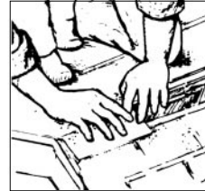
3. Let top course of shingles lay over unslotted portion of ridge (ends) to form one thickness.
