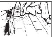
7. Use power saw to cut through roof sheathing along chalk lines. Set depth to avoid cutting into rafters. Watch for nails.
